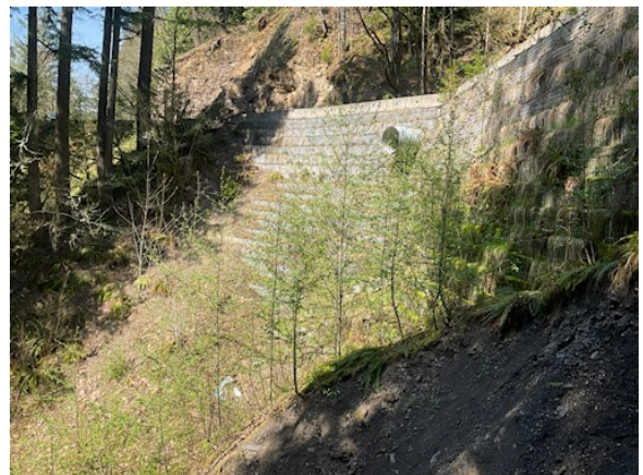
Town side of wall performing well
