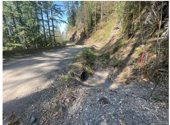
Woods culvert has limited flow. Pool from town culvert should get here.
